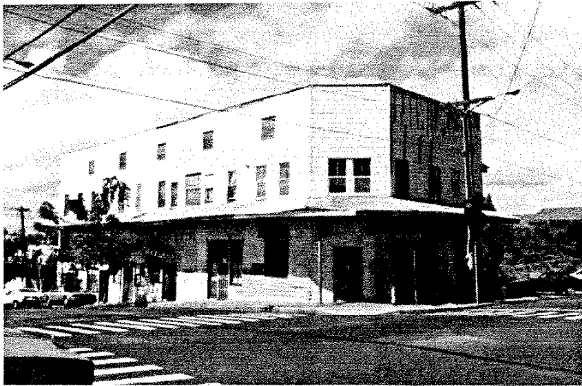
An existing building on the corner of Waipahu Street and Waipahu Depot Road which has probably outlived its useful life.
