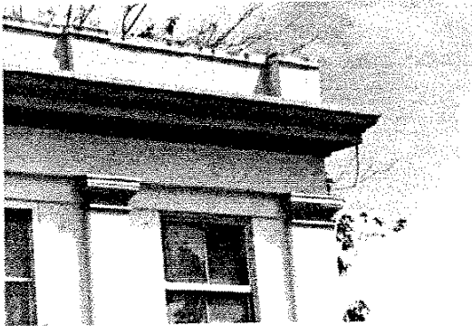
Roof parapet and cornice details of the old Waipahu Store.
